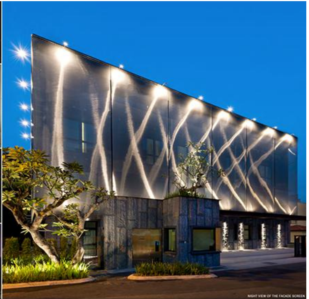
NIGHT VIEW OF THE FACADE SCREEN
