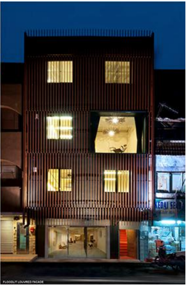
FLOODED LOUVERED FACADE
