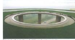
Rainwater is collected at the roof, which goes down to a reservoir.
