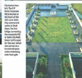
Investment in renewable energy was RM400,000, with savings of RM21,264 per year and return on investment in 16 years. Some RM300,000 was invested in rainwater harvesting resulting in annual savings of RM10,444 with return on investment in 24 years.
